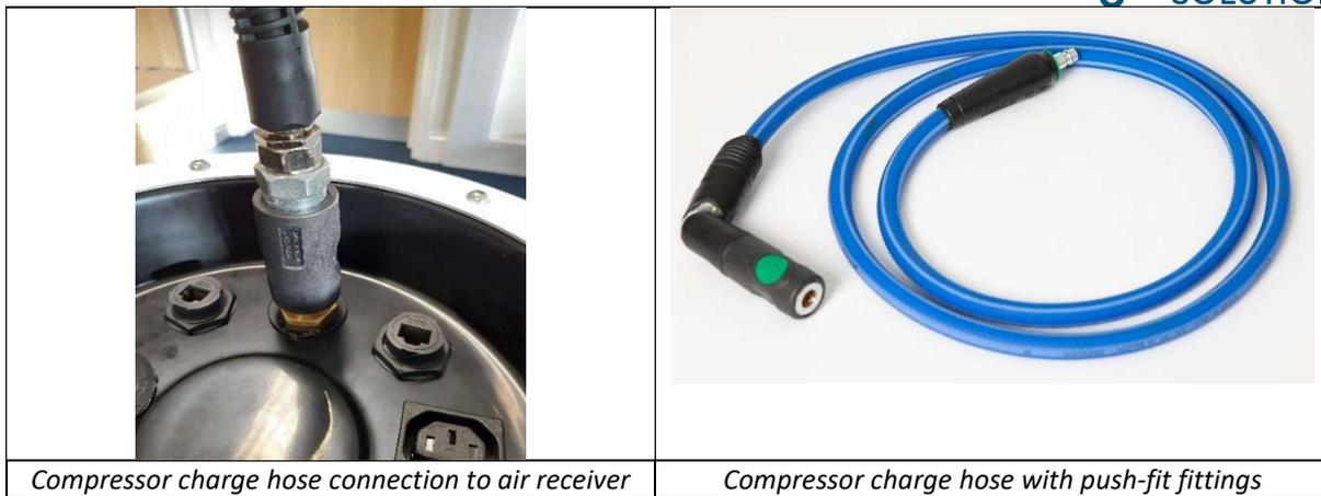
**NOTE: FOR THIRD PARTY SUPPLIED COMPRESSORS, ENSURE YOUR COMPRESSOR IS SET TO CHARGE TO 9-10BAR TO ENSURE THE TANK'S SAFETY VALVE IS NOT TRIGGERED.**
