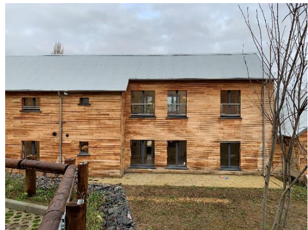
Low rise block of Passivhaus flats
