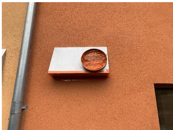
MVHR units switched off with both inlet and exhausts either sealed internally or externally
