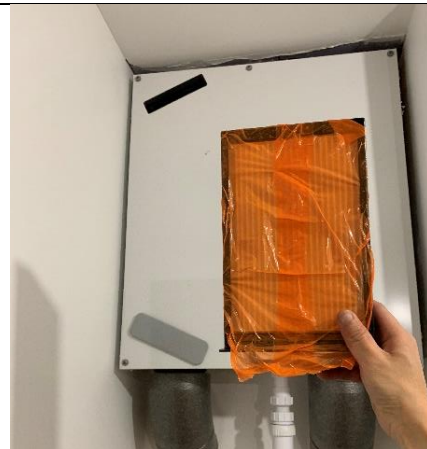
MVHR units switched off with both inlet and exhausts either sealed internally or externally
