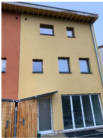
3 Storey house in Colchester
