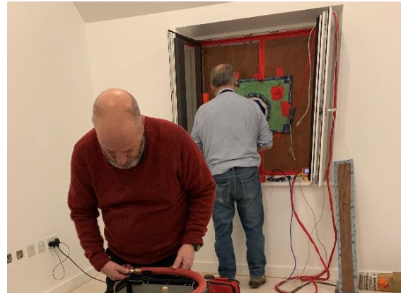
Blower door fan mounted and sealed in a panel cut to the size of the window opening
