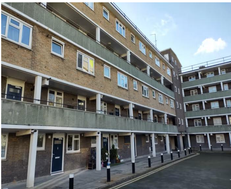
Treadgold House on the Lancaster West Estate before retrofit works
