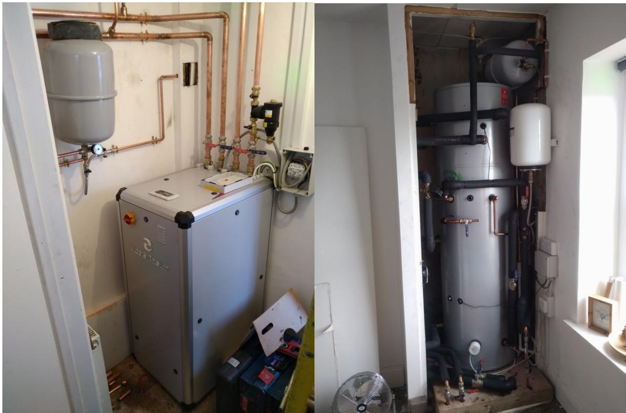
Figure 6: MasterTherm AQ37i1 GSHP (left) and Joule 300l DHW + 90l buffer cylinder (right) in-situ
