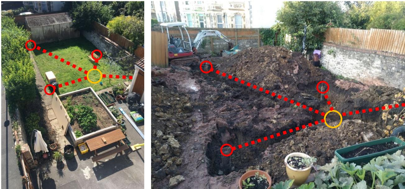
Figure 4: Locations for Boreholes (red), Manifold (orange) and Lateral Pipework (red-dash) in Rear Garden<sup>9</sup>
