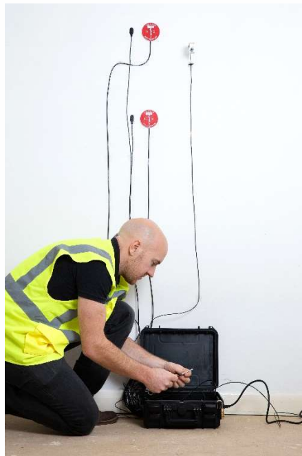
Figure 24: Heat flux plates being installed on a wall.
