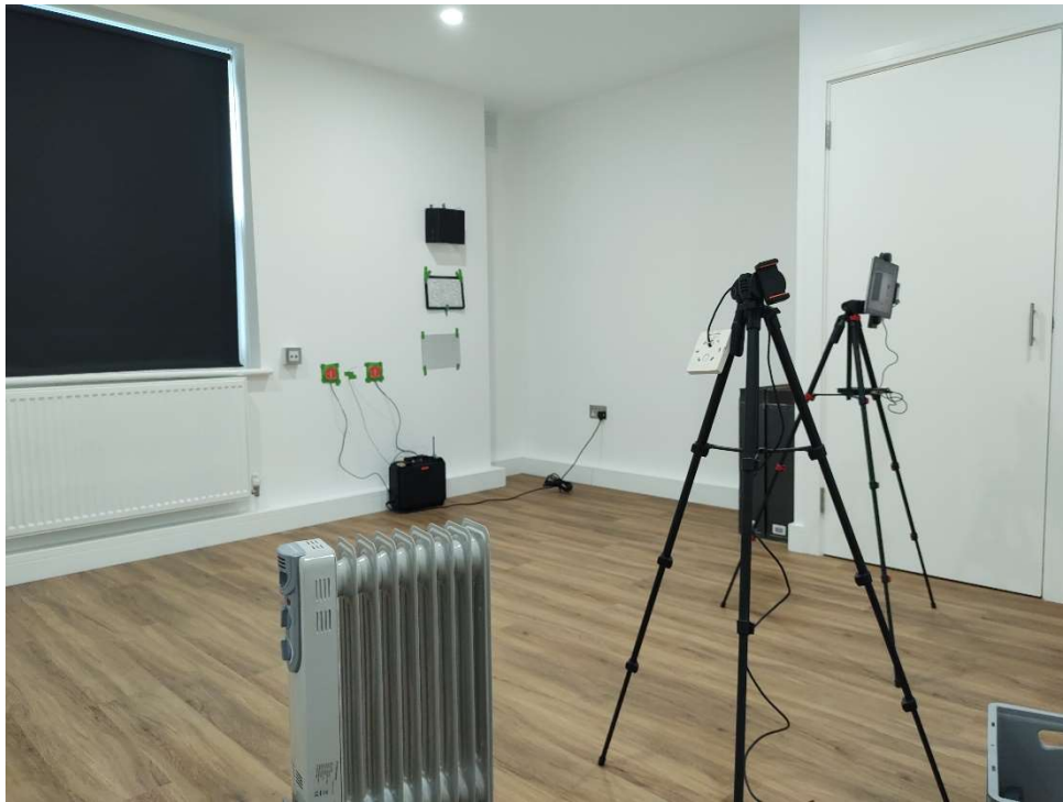
Figure 7: An example field trial installation with heat flux plates adjacent to an uncovered section of wall where the Heat3D measurement was taken.
